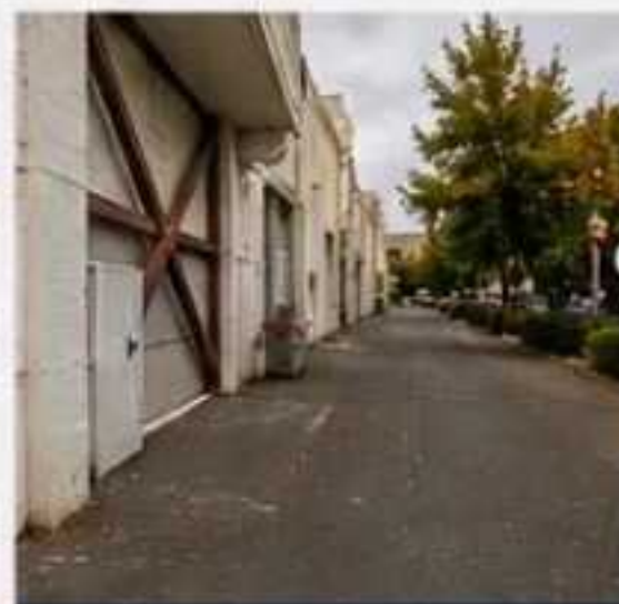
EXISTING CONDITIONS - MID ALLEY
